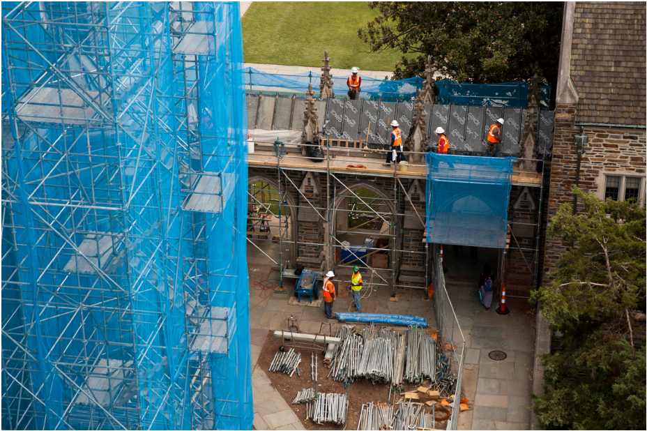
Restoring the Roofs outside Duke University Chapel.
