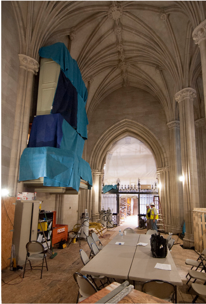
Work inside Memorial Chapel.
