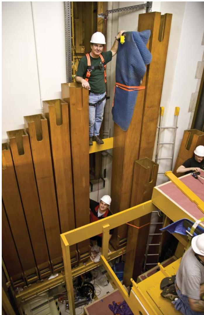
*Phil Carpenter, Head of Field Operations for Foley-Baker, Inc. stands admist large wooden pipes being installed after reconditioning.*
