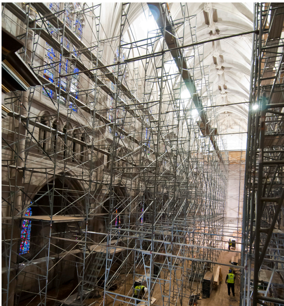
Scaffolding with platforms have been built so crews can reach the Chapel ceiling Please continue to pray for the Chapel and all those working on its restoration. Photo Credit: Ray Walker, Duke Facilities architect/project manager.
