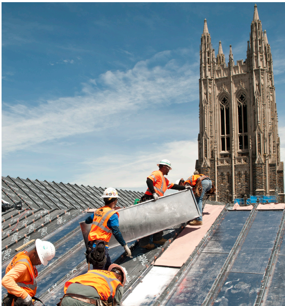
Crews work to remove and replace lead-coated copper roofing panels. Please continue to pray for the Chapel and all those working on its restoration. Photo Credit: Ray Walker, Duke Facilities architect/project manager.
