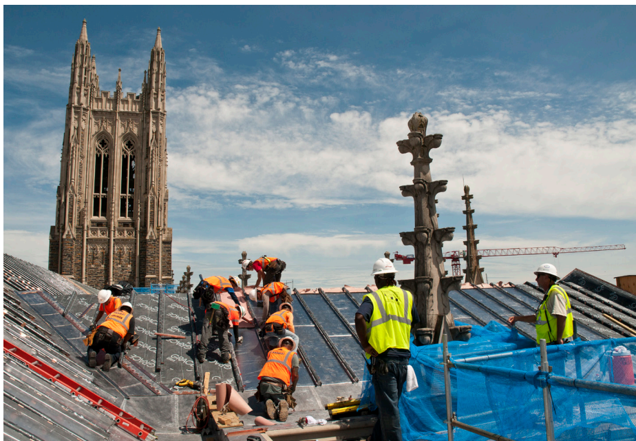
Crews work to remove and replace lead-coated copper roofing panels. Please continue to pray for the Chapel and all those working on its restoration. Photo Credit: Ray Walker, Staff Architect and Project Manager, Duke Facilities Management
